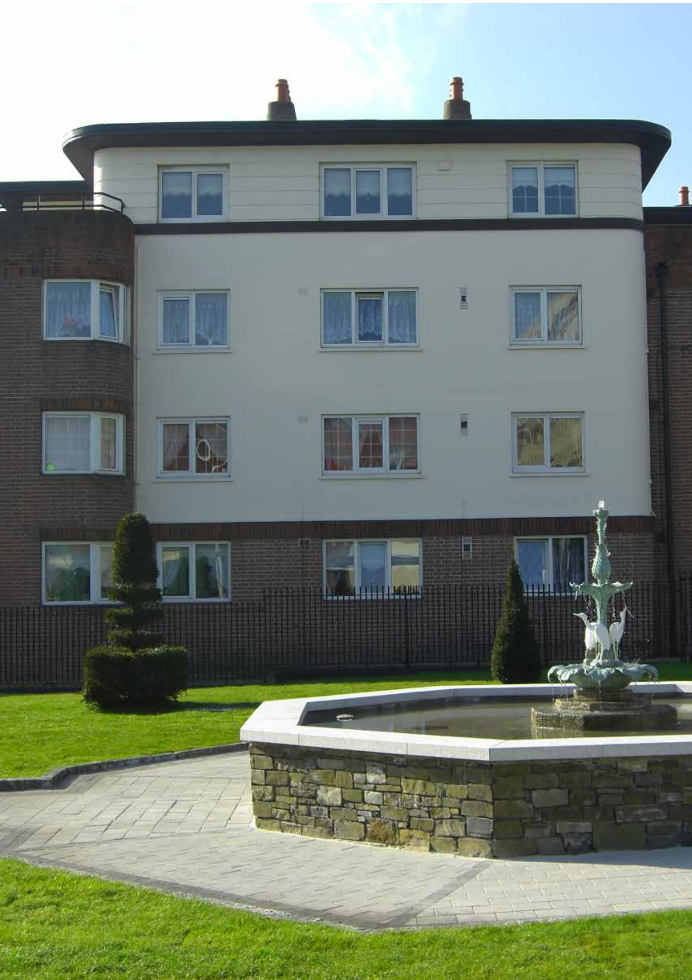
Chancery Street House and Chancery Park
